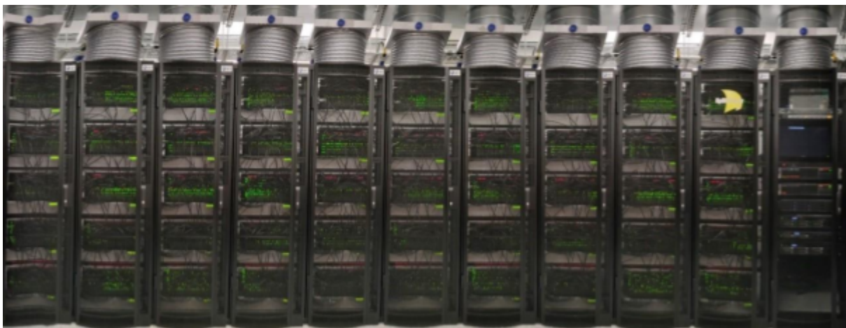
Figure 1: A 10 cabinet machine, wired together (Note: the 11th cabinet in the picture contains servers for handling jobs sent to the machine).
